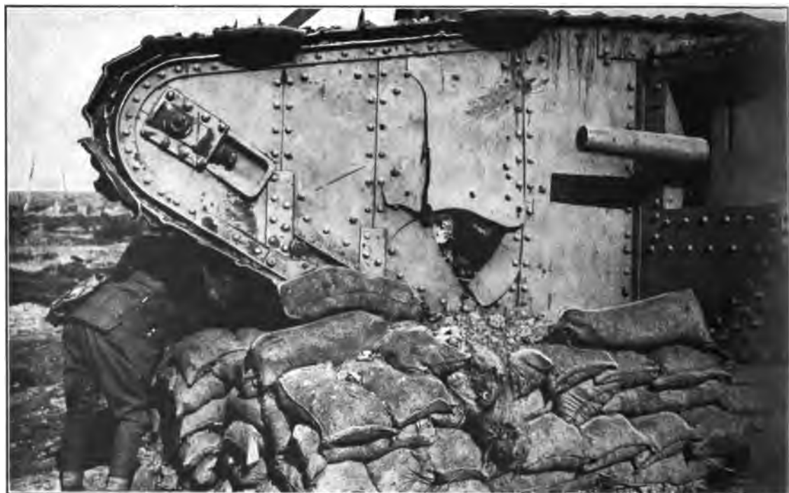
A DERELICT TANK USED AS THE ROOF OF A DUGOUT
